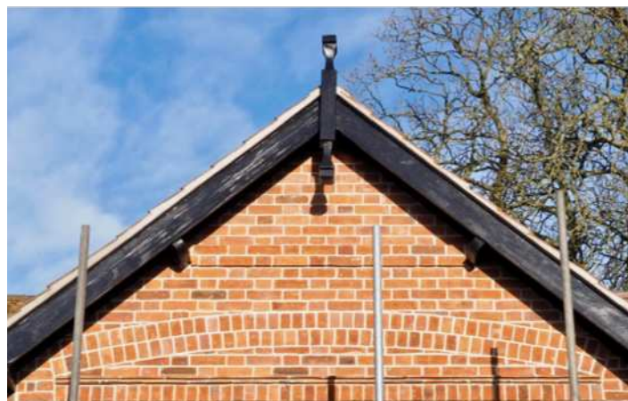
Front, first floor elevation which David Ruse has re-bricked in great detail
