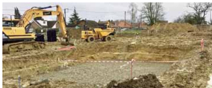
Digging the large hole for the 'attenuation tank'
