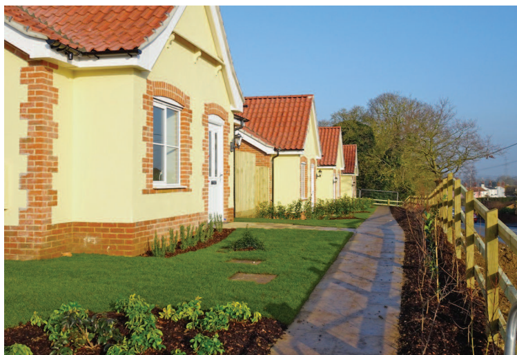
The two bedroom bungalows facing Ipswich Road, Grundisburgh.
